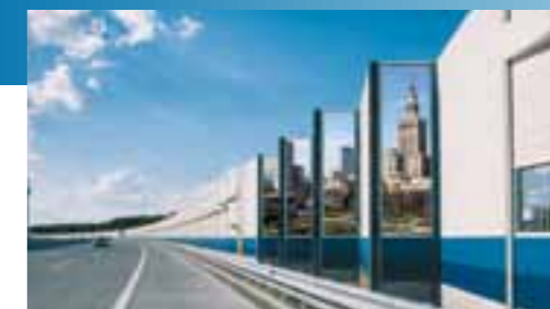
Noise protection wall with glass panels and digital design
