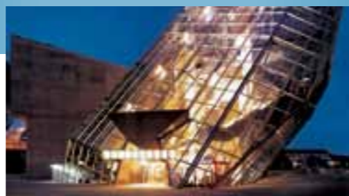
UFA-Palast Dresden, individual post-and-beam construction
