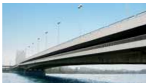
Reichsbrücke, Vienna, ALUMERO Bond composite panels
